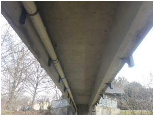
VIEW FROM BELOW - LOOKING EAST
