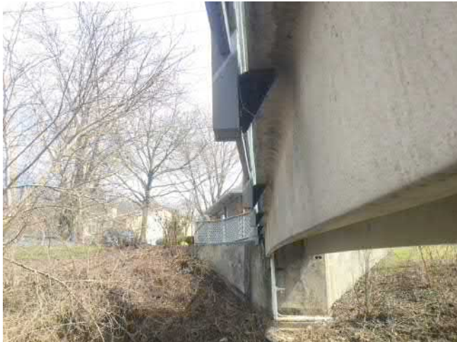
NORTH SIDE OVERHANG
